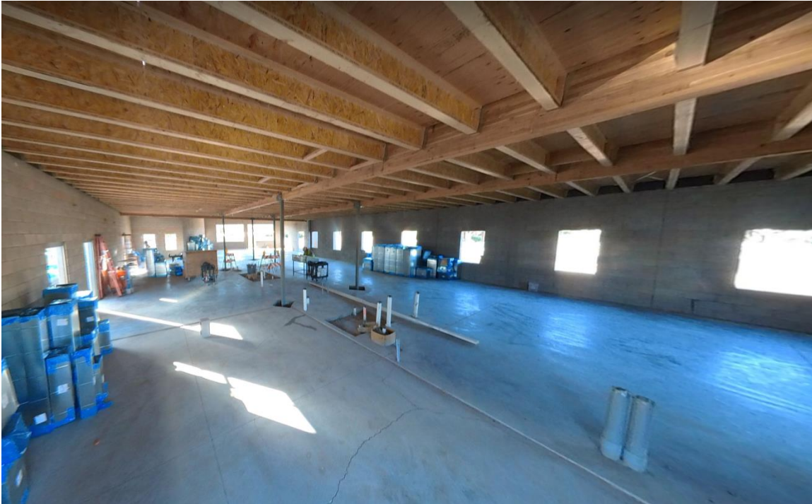
Living quarters at the new Station 152 (early May 2023)
